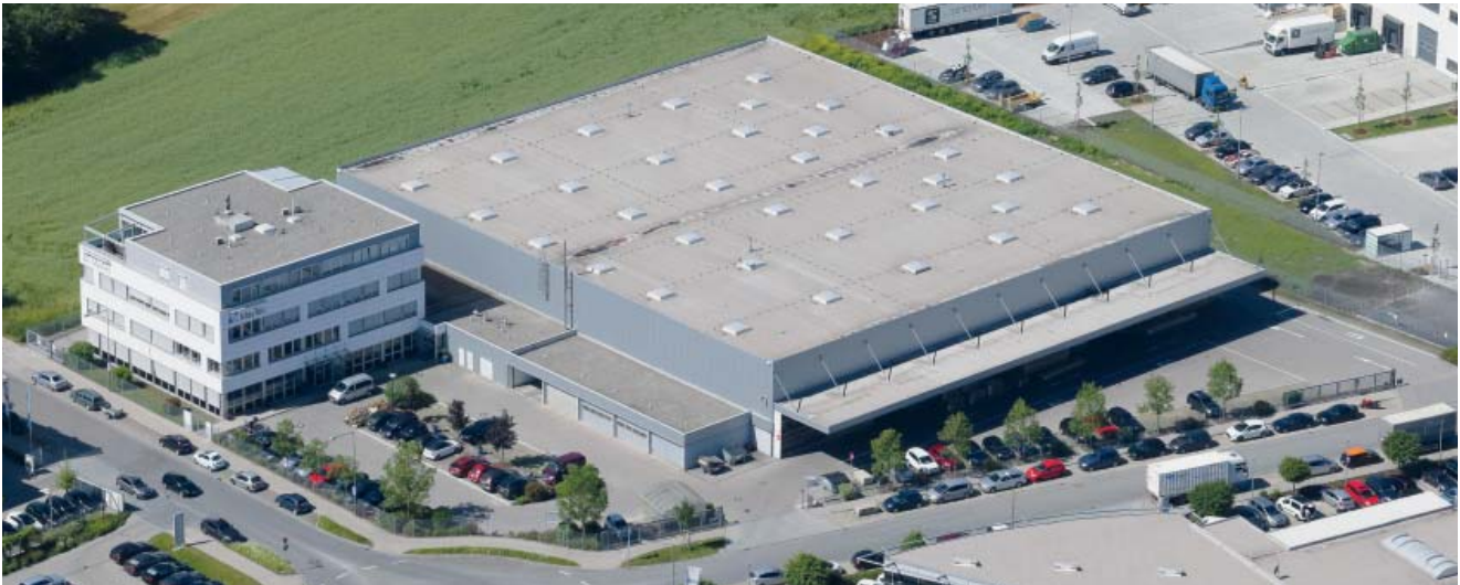
MayTec GmbH plant in Dachau
